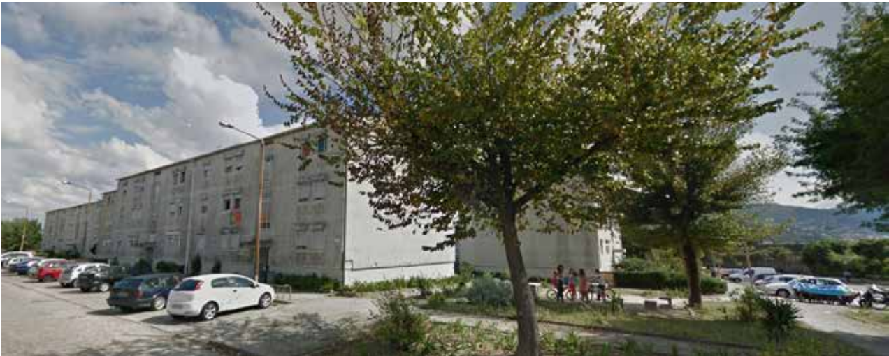
Ringe's Housing Complex
